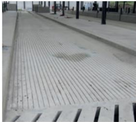
Grooved concrete flooring is used successfully in the dairy sector
