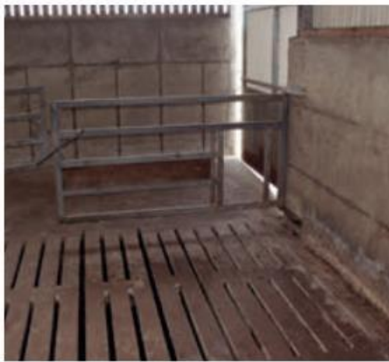
Slatted floor without rubber matting
