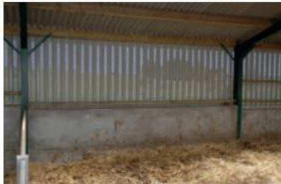
Perforated wall cladding
