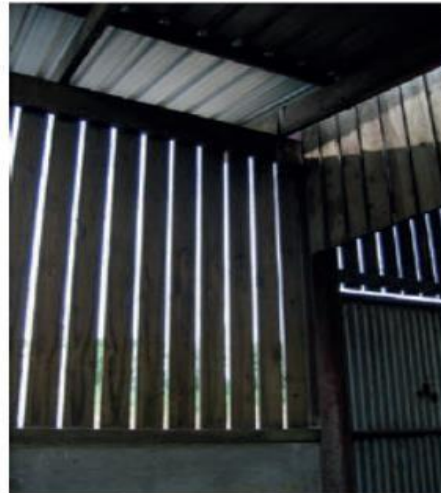
Spaceboard with a simple additional inlet area allows fresh air to enter
