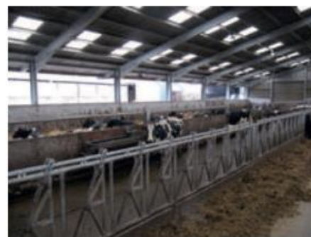
Feed barriers with locking yokes
