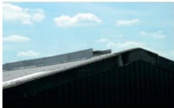
A covered open ridge
