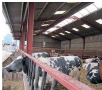
The addition of a light ridge will improve ventilation and increase the amount of natural lighting
