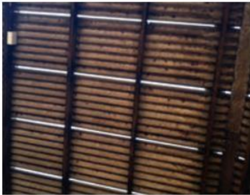
A slotted roof is good where animals are housed all year
