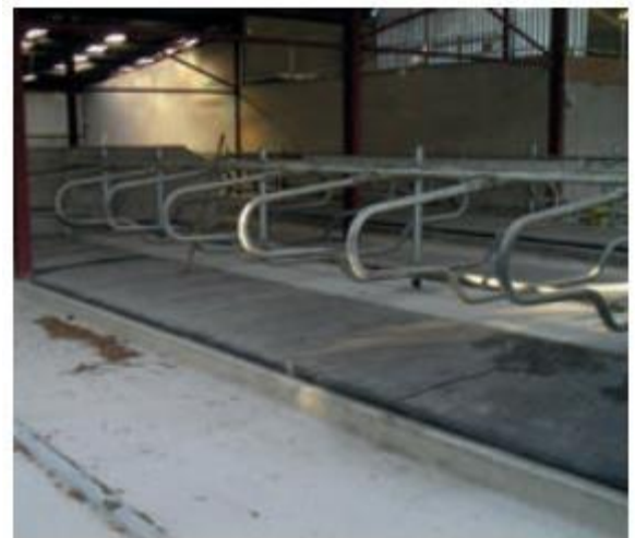
Cubicles with rubber matting
