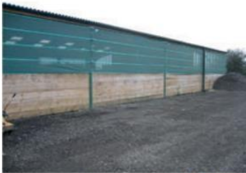
Timber sidewall with ventilated cladding delivers clean fresh air into the building
