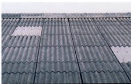
Slotted roof made of fibre cement profiled sheeting
