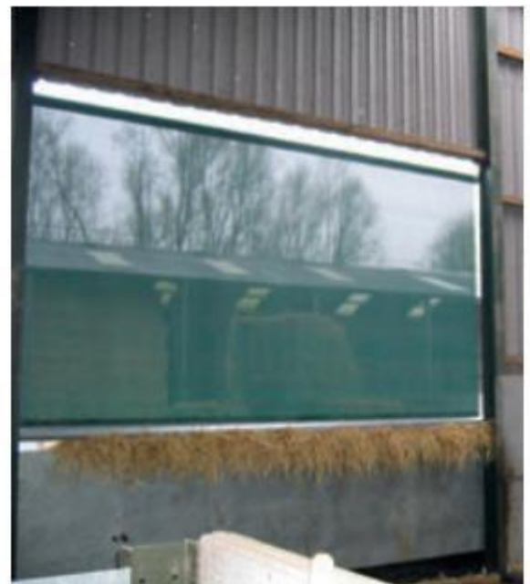
A ventilated roller blind offers protection against draughts
